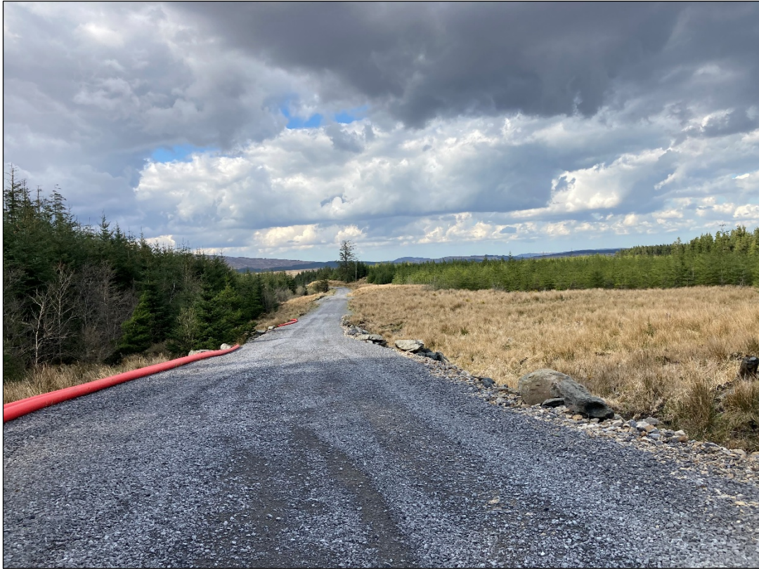
View North along Main Spine Road
