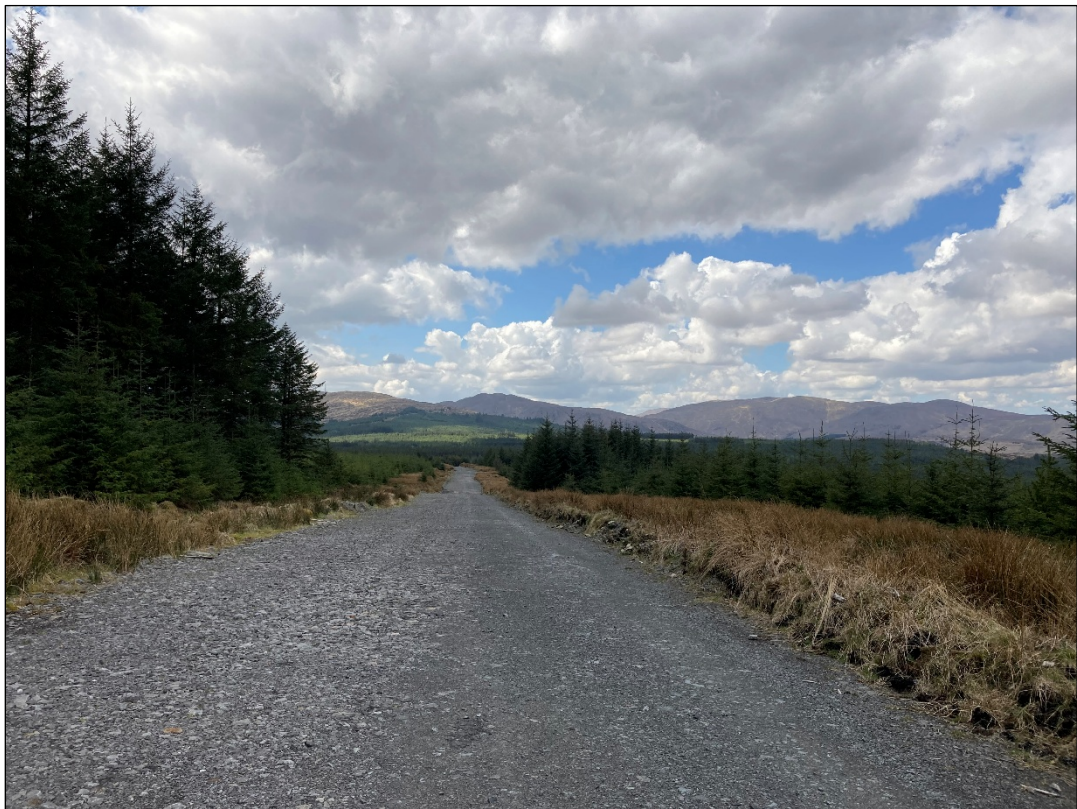
View West along founded access road between T11 and T12
