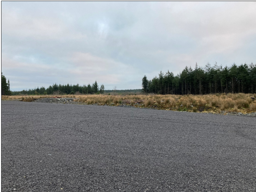
View of hardstand at T11
