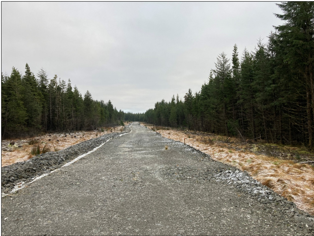
Section of Floating Road to T04
