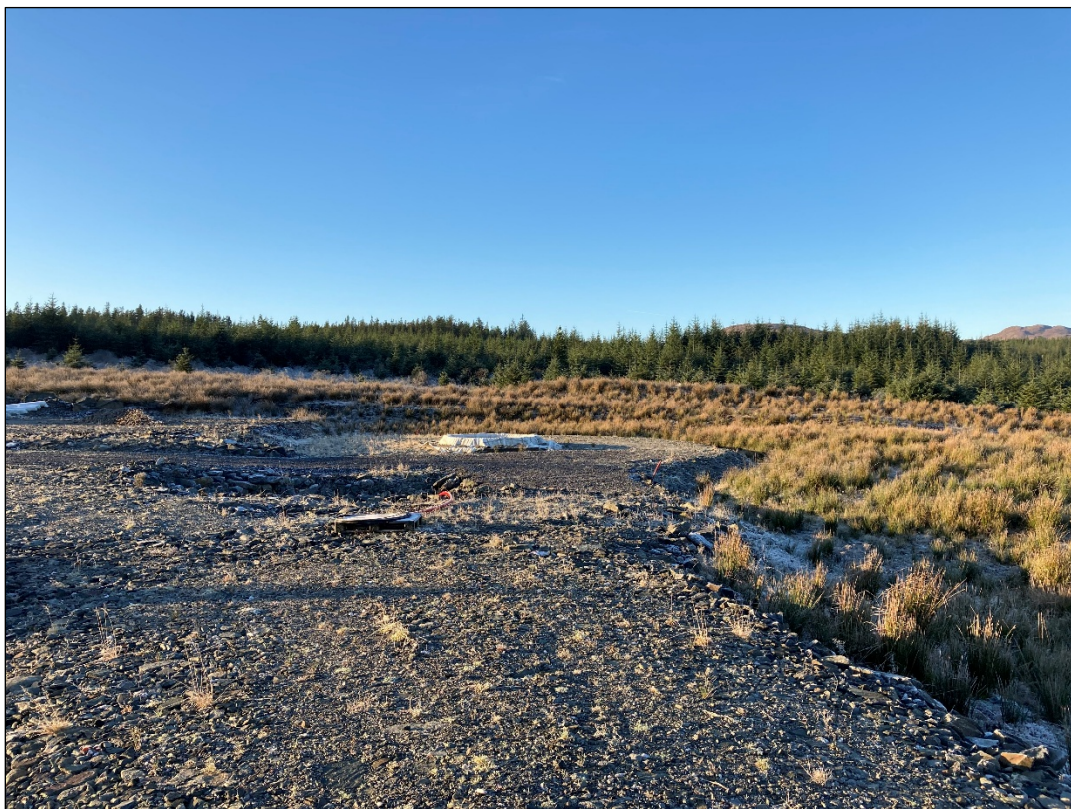
Turbine base and hardstand, T14
