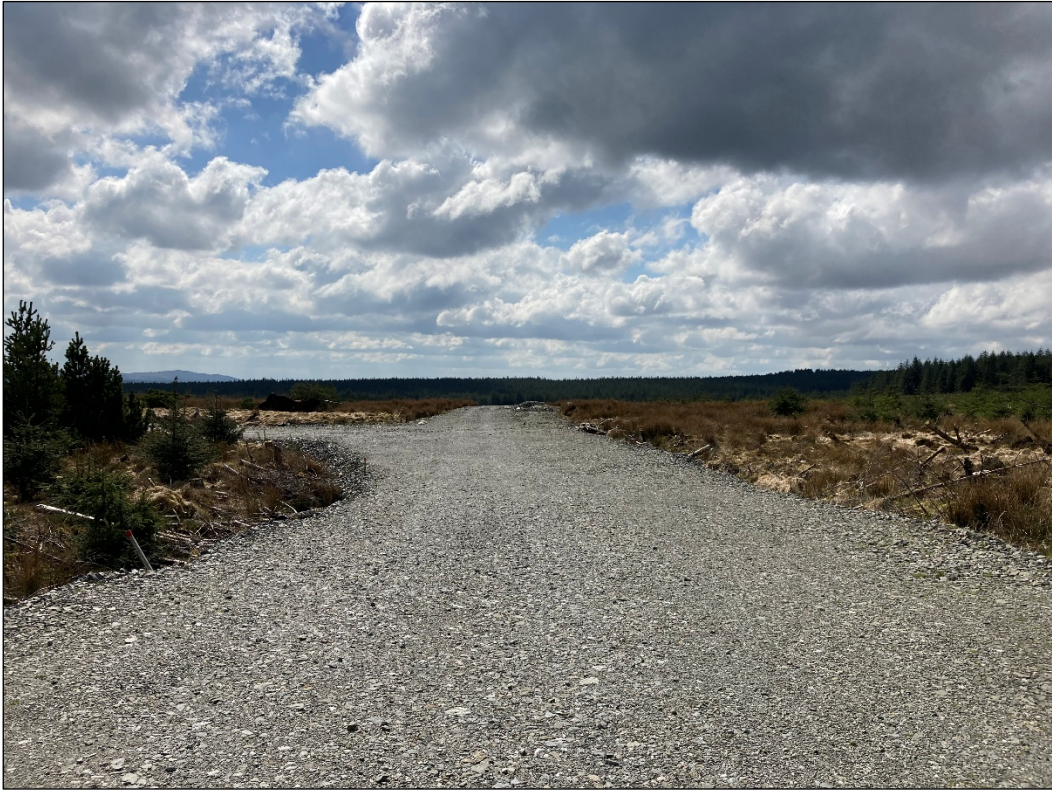
Looking south at section of floating road at Junction to T01 and T04
