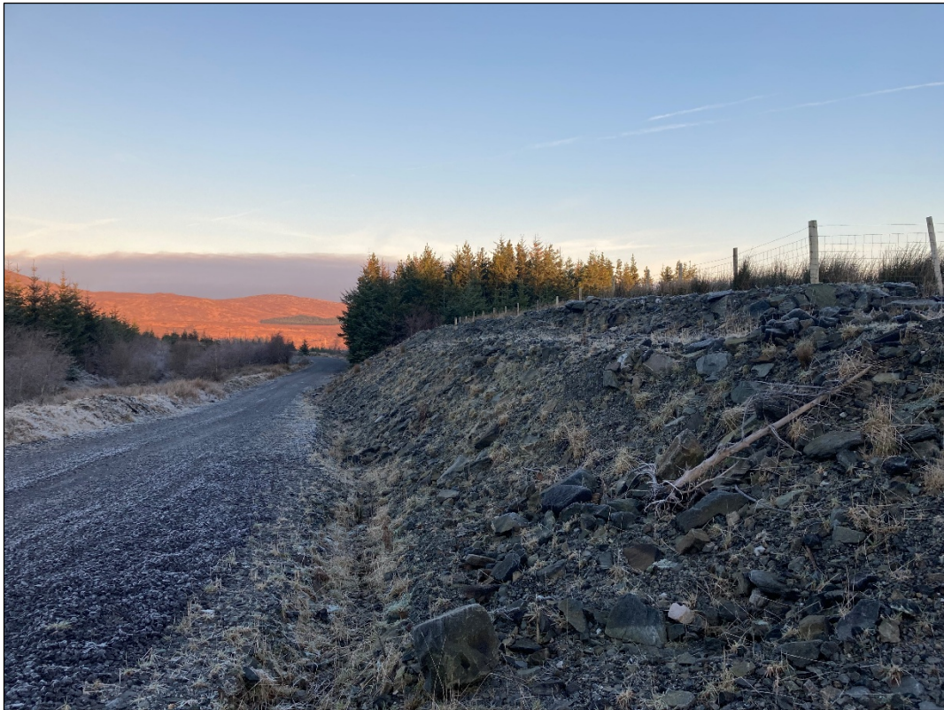
View of berm at Peat Cell at Substation
